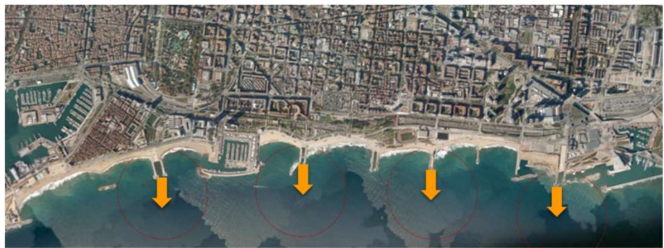
Sewer overflow points on the beaches of Barcelona
