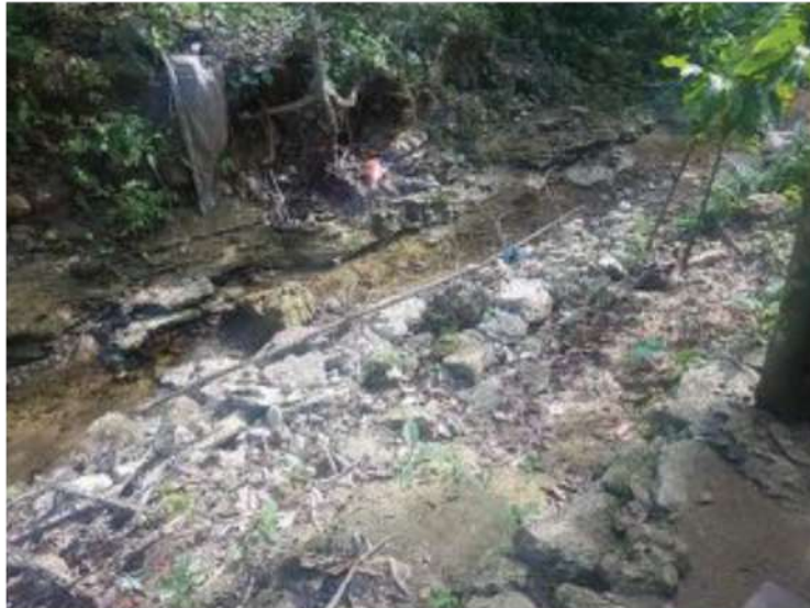
Figure 36. Current Condition of the Waterway in Brgy. Malinao last 13 January 2020
