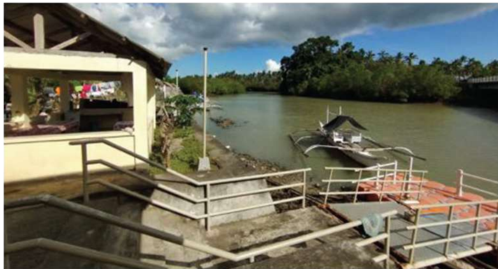
Figure 33. Firefly Watching Visitor Center and Landing Area
