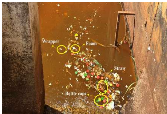
Figure 9.2. Trapped Plastics in the Preliminary Screening Process of a Wastewater Treatment Plant in the Lao PDR
