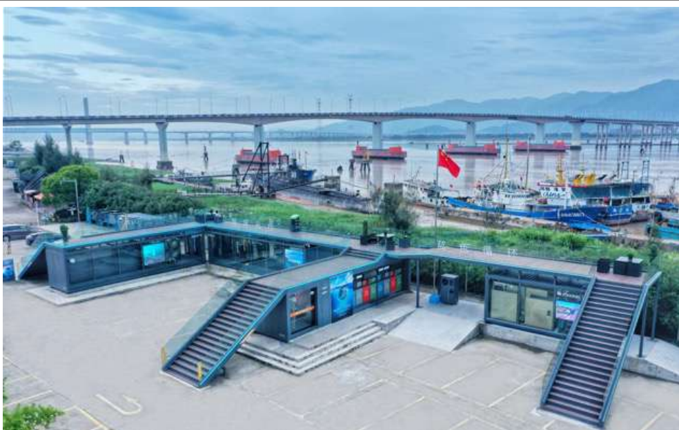
Figure 20.3. Ocean Cloud Warehouse Operating at Jiaojiang Central Fishing Port, Taizhou, Zhejiang
